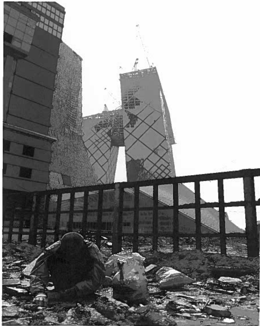
CCTV, Beijing. Photo by the author
