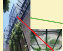
Steel frame mounted green screen panels provide a tall vertical landscape element from pedestrian level to upper level balconies of the outdoor sitting area.
